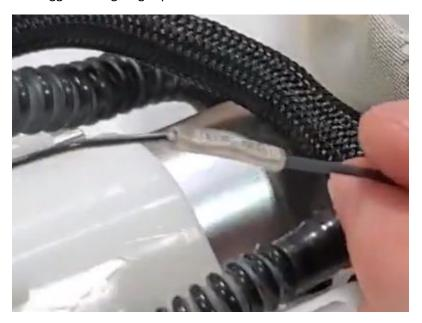
Slide the shrink tube over this metal crimp once complete and shrink into place using a heat gun.
